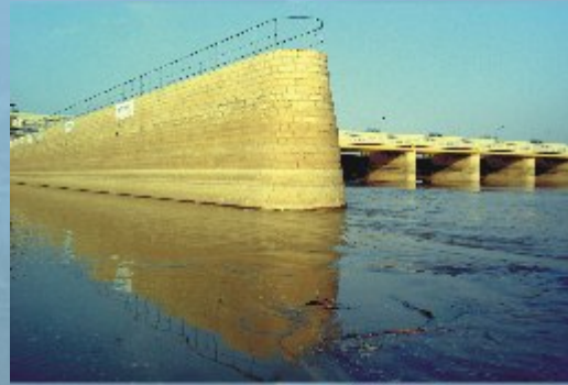
Different water levels visible on barrage walls.
