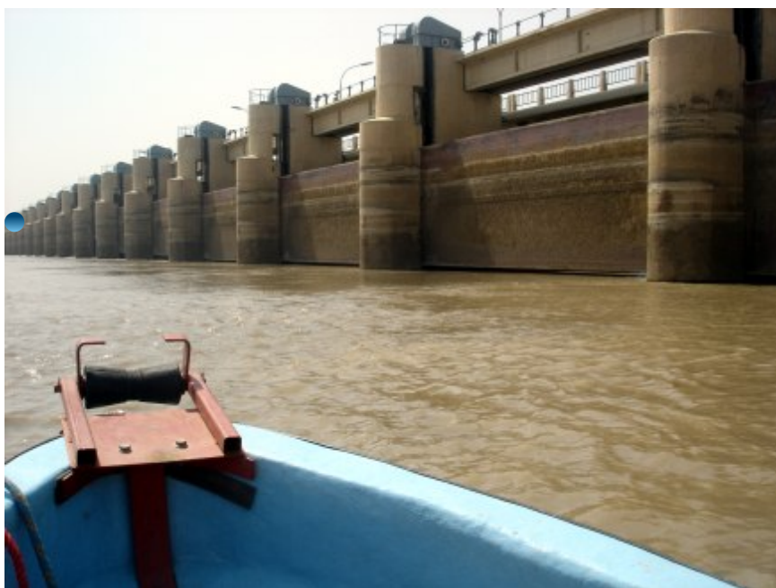
A View of the Barrage gates.
